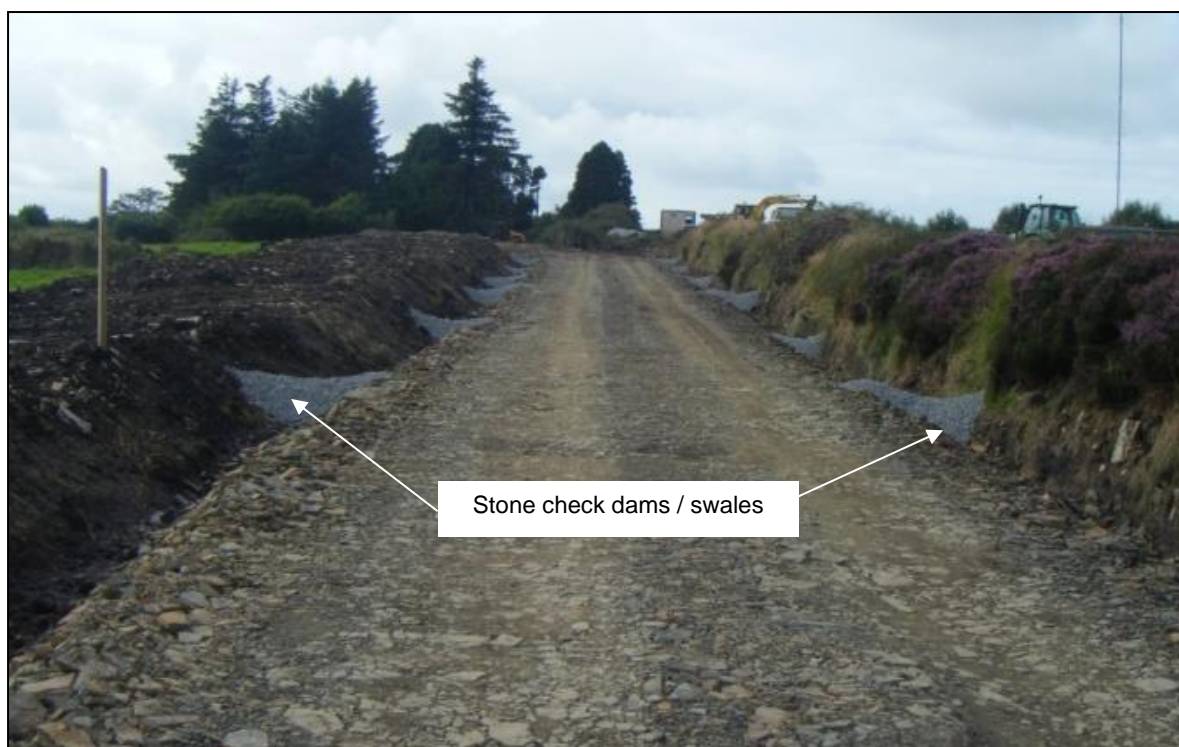
Figure 5 – Example of check dams along roadside drainage channels
