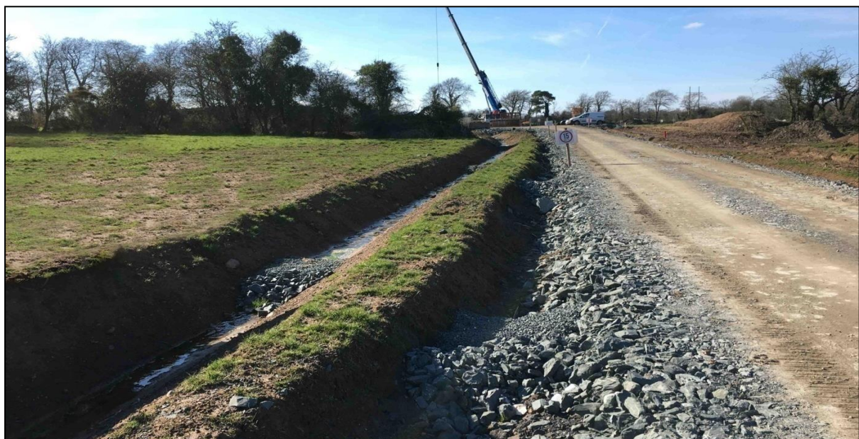
Figure 2 – Separation of clean and dirty water drainage on wind farm site
